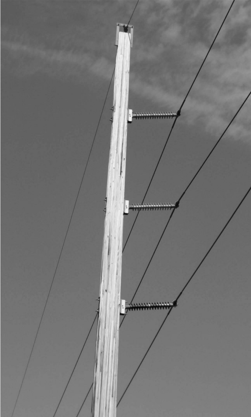
Figure 1.7 Laminated Wood Pole.
