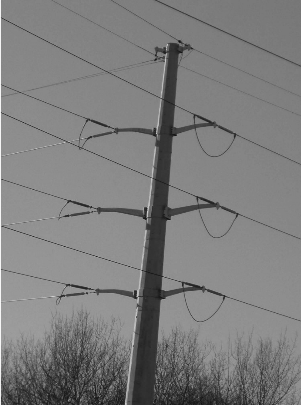
Figure 1.4b Steel Pole Deadend – Tangent and 90 degrees.
