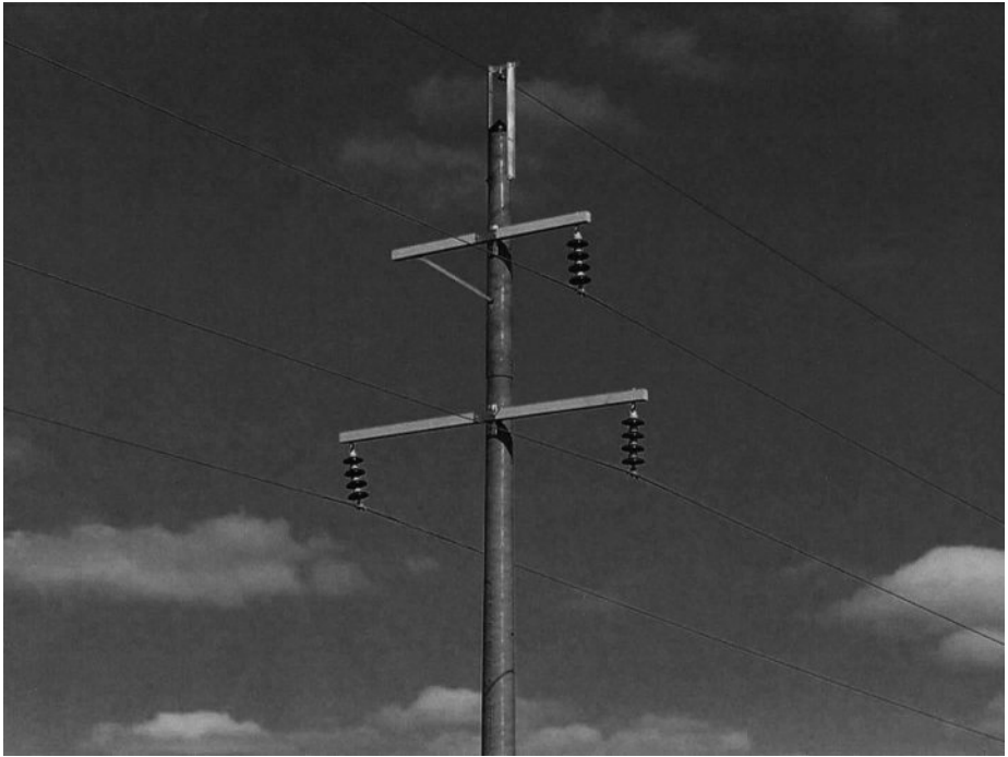
Figure 1.8a Composite Pole with Cross Arms.
