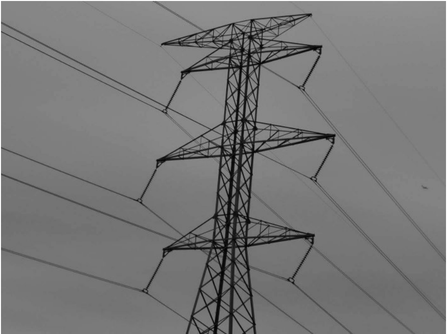
Figure 1.5 Lattice Tower.
