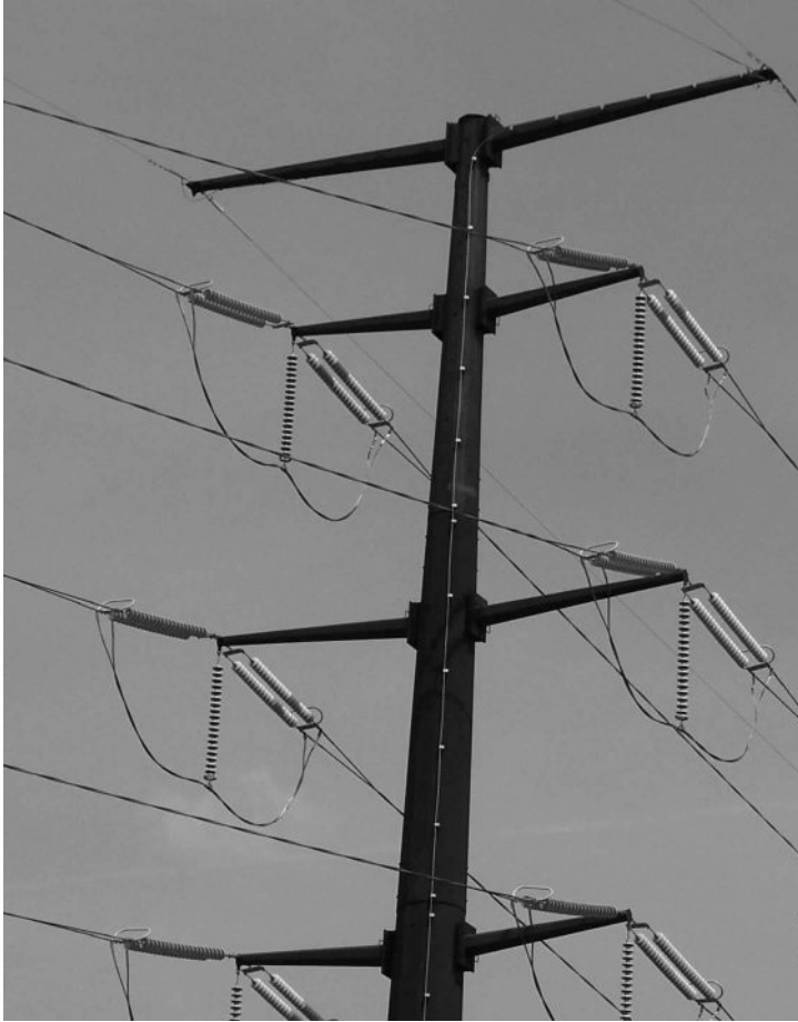
Figure 1.4c Steel Pole – Deadend Tangent.
